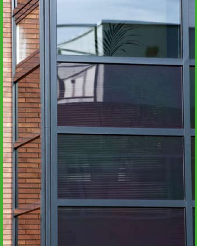
Detail van de panelen in Roomburg
